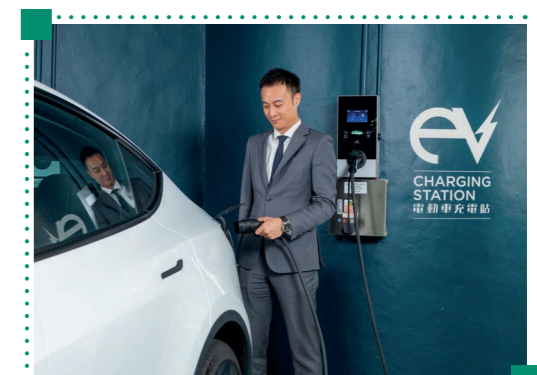
Enabling sustainable mobility with new electric vehicle charging points
