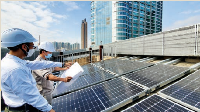
Installation of Solar Panels
