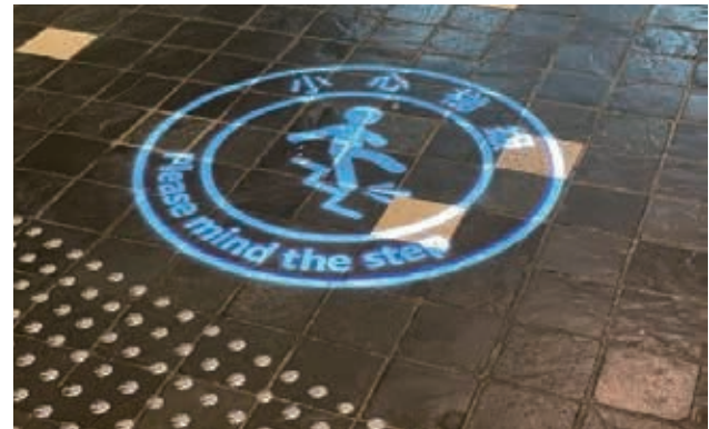
Motion projection lightings for falling accident prevention
