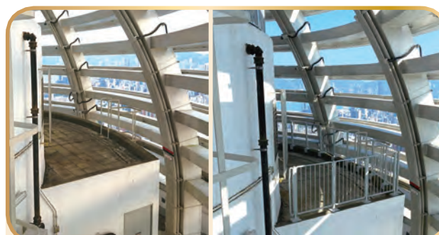
Protective Barrier on Roof Floor
