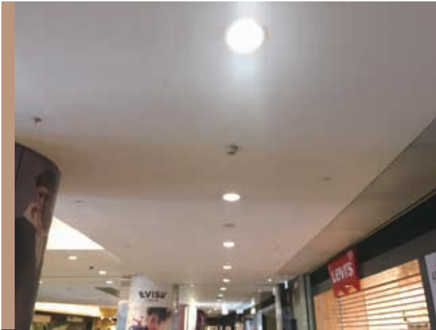
Retrofit of Metal Halide to LED Lights
