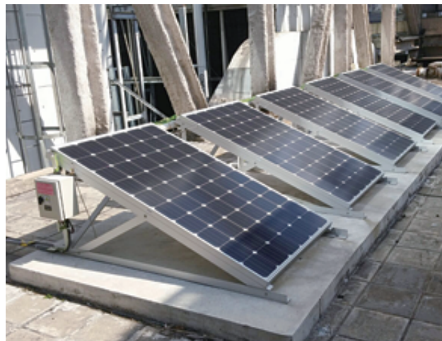
Installation of Solar Panels
