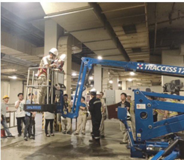
Field Demonstration of Using Aerial Working Platform
