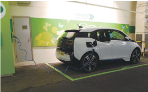
Upgrade of EV Charging Station
